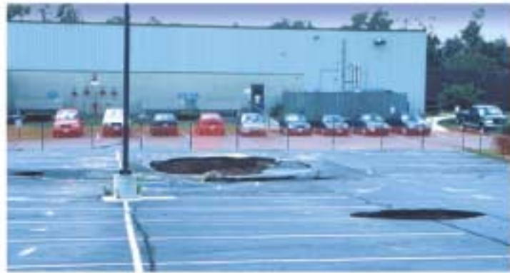
Fig. 1. Sinkholes in collapsed parking area, Frederick, MD. Sinkholes form in carbonate areas as the dissolving and weakening of bedrock cause it to collapse.
